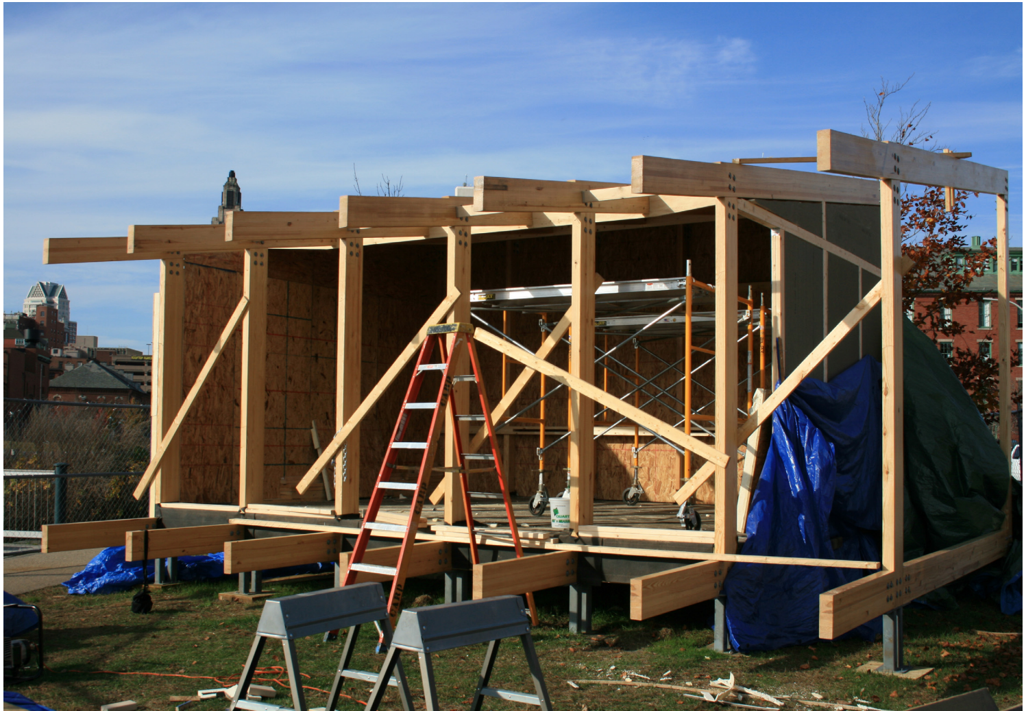
Frame with recovery-board sheathing between ribs: View looking north
