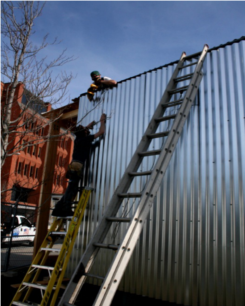
Above: Corrugated metal sheathing installed on North facade of Solar Pavilion
