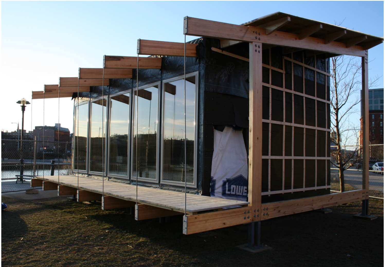
Sealed, glazed enclosure: View looking west
