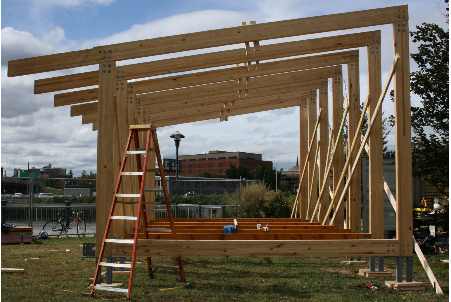
Completed erection of Glulam ribs: View looking west
