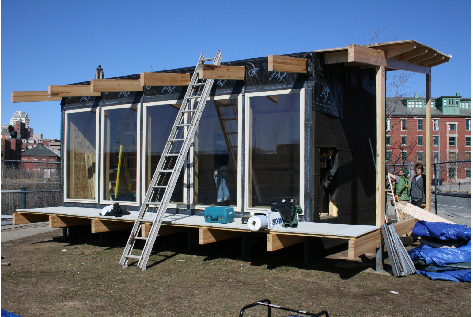
Framed & Sealed Enclosure with southern glazing; View looking north
