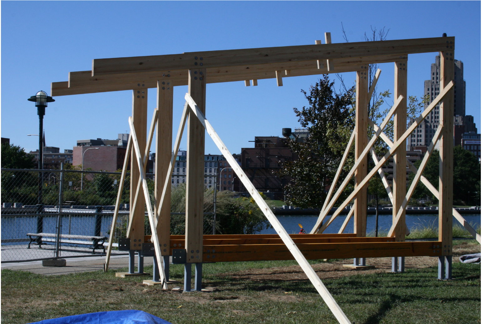
Installation of first three Glulam ribs in footings: View looking west
