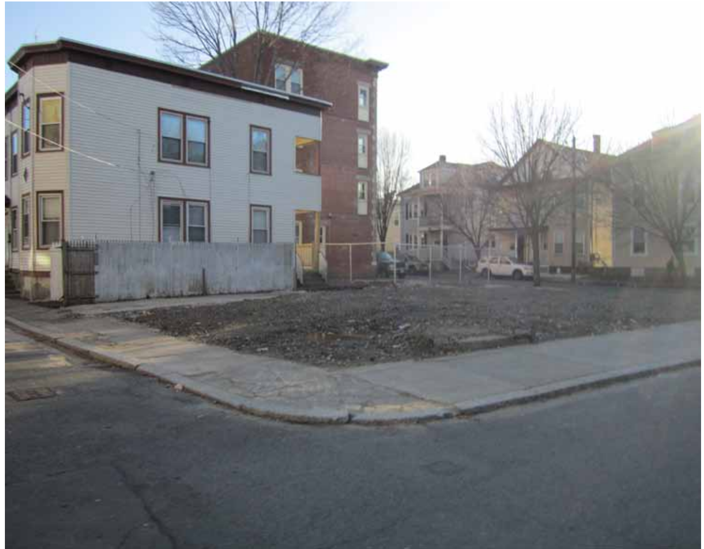
Existing Conditions at Palmer Street Property
